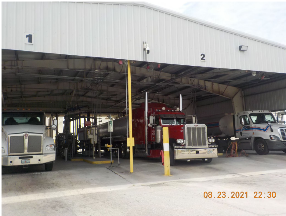
Photo #1 – Tanker truck loading rack (TTLR) area.
