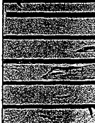
Photograph of a house in the Middle West; low-grade paint only one year old. It has gone "all to pieces." This surface must be burned and scraped before it can be repainted.
