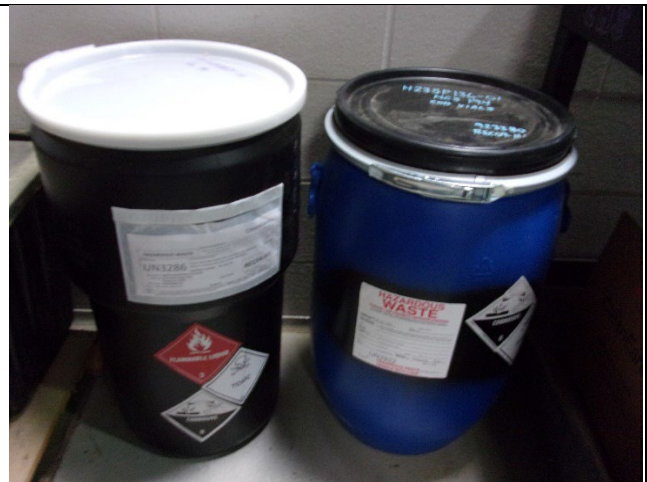
Figure 2: July 11, 2023, 9:24 AM WMF: Room 214-R Reactives Two (2) 5-gallon containers with hazardous waste label, accumulation start date, and indication of the hazards of the contents.
