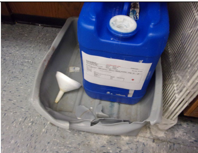
Figure 19: July 12, 2023, 9:14 AM Dabney Hall: Room 847 Damaged secondary containment bin.
