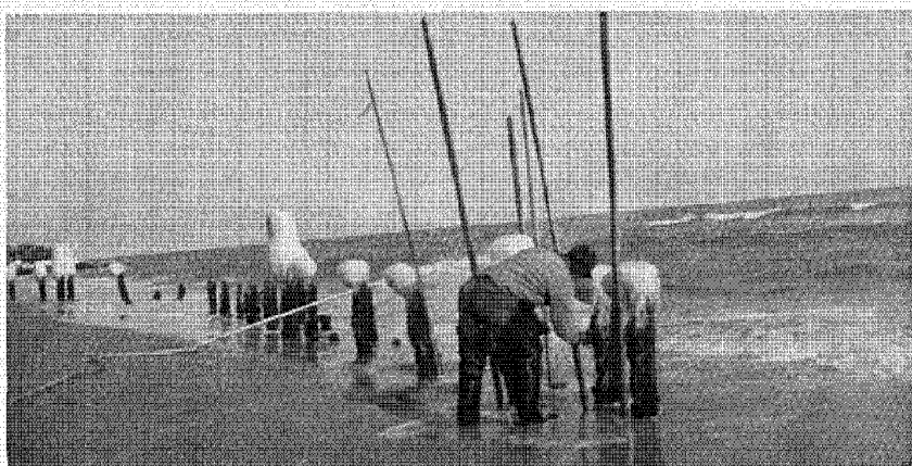
A row of charges in place and ready to be fired. The ice-capped pilings show the conditions under which the work was done
