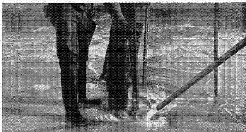
A water jet was used to displace sand so that the dynamite cartridges, tied to the end of a lath, could be lodged, at the required depth, against the pile to be cut off
