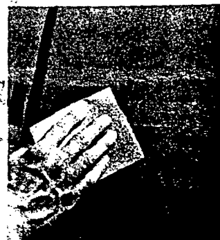
After drying, cement is sandpapered evenly, assuring a smooth surface for any decoration.
