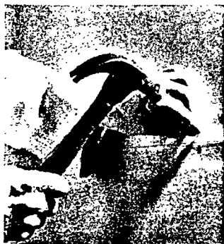
When the sheets are nailed in place, the recessed edges form a channel at each joint.
