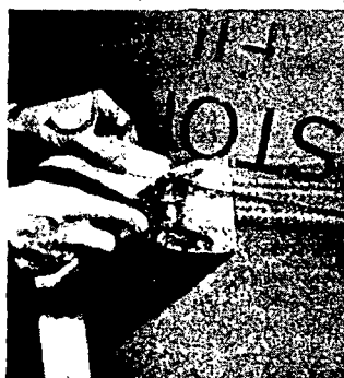
Perf-A-Tape, a strong, perforated fiber tape with chamfered edges is embedded in the cement.
