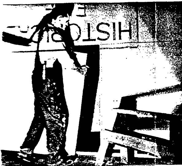
ReCESSED-EDGE SHEETROCK being applied horizontally—at right angles to framing—to give increased bracing strength.
