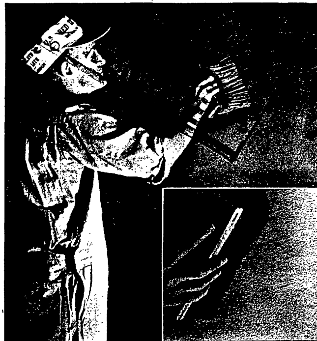
(Above) Textone being applied over Recessed-Edge Sheetrock-Perf-A-Tape wall. Insert shows how fine Colonial stippled effect is obtained. (Below) The finished job—walls of Recessed-Edge Sheetrock, joints reinforced and hidden with Perf-A-Tape, decorated with Textone and Texolite.
