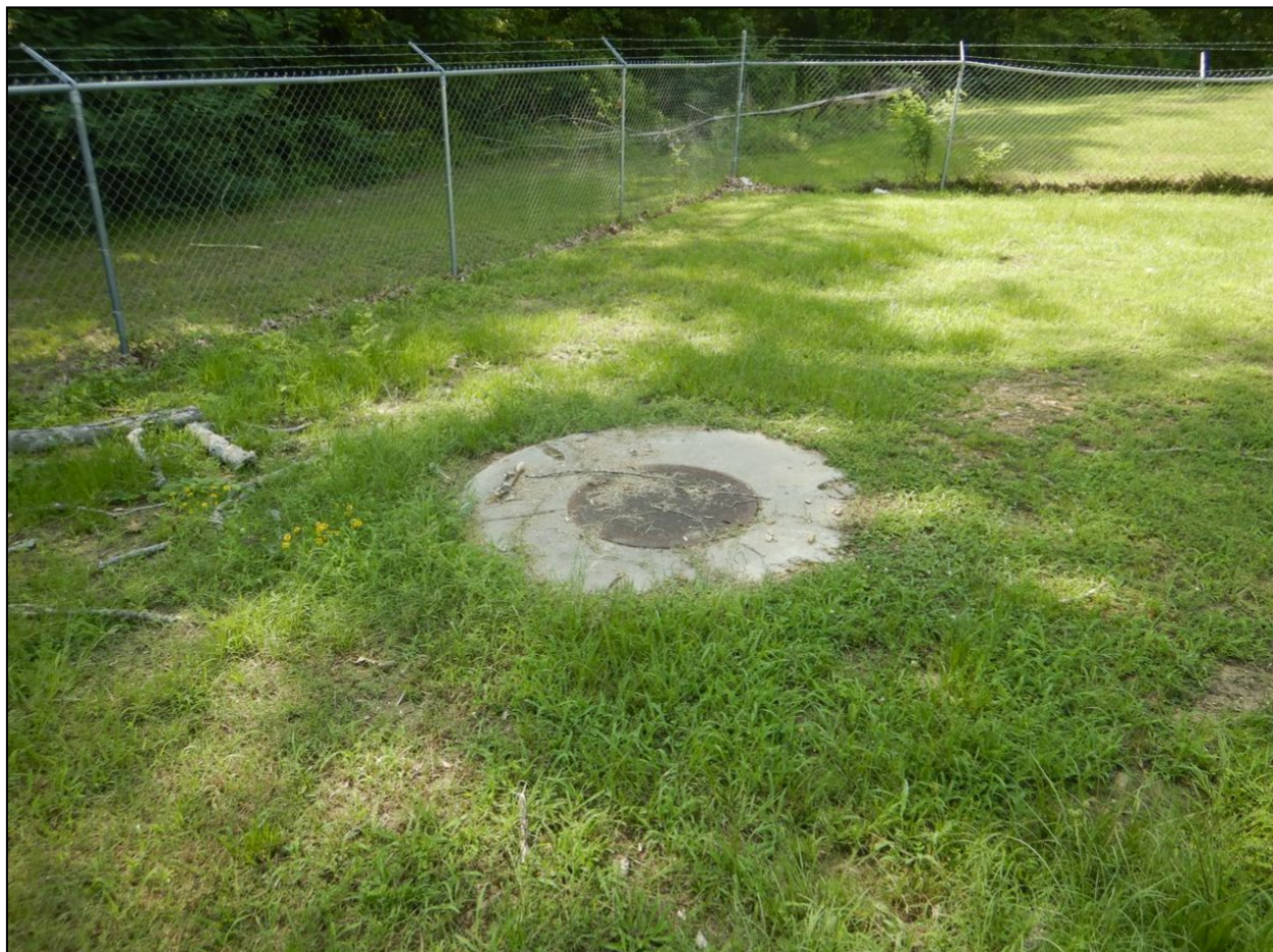
Photograph 5. Chemical Addition Manhole, WTP #01 View of the chemical addition manhole located outside of WTP #1. The manhole leads to the raw water influent pump line. The System Manager stated that coagulant and sodium permanganate were added at this point.
