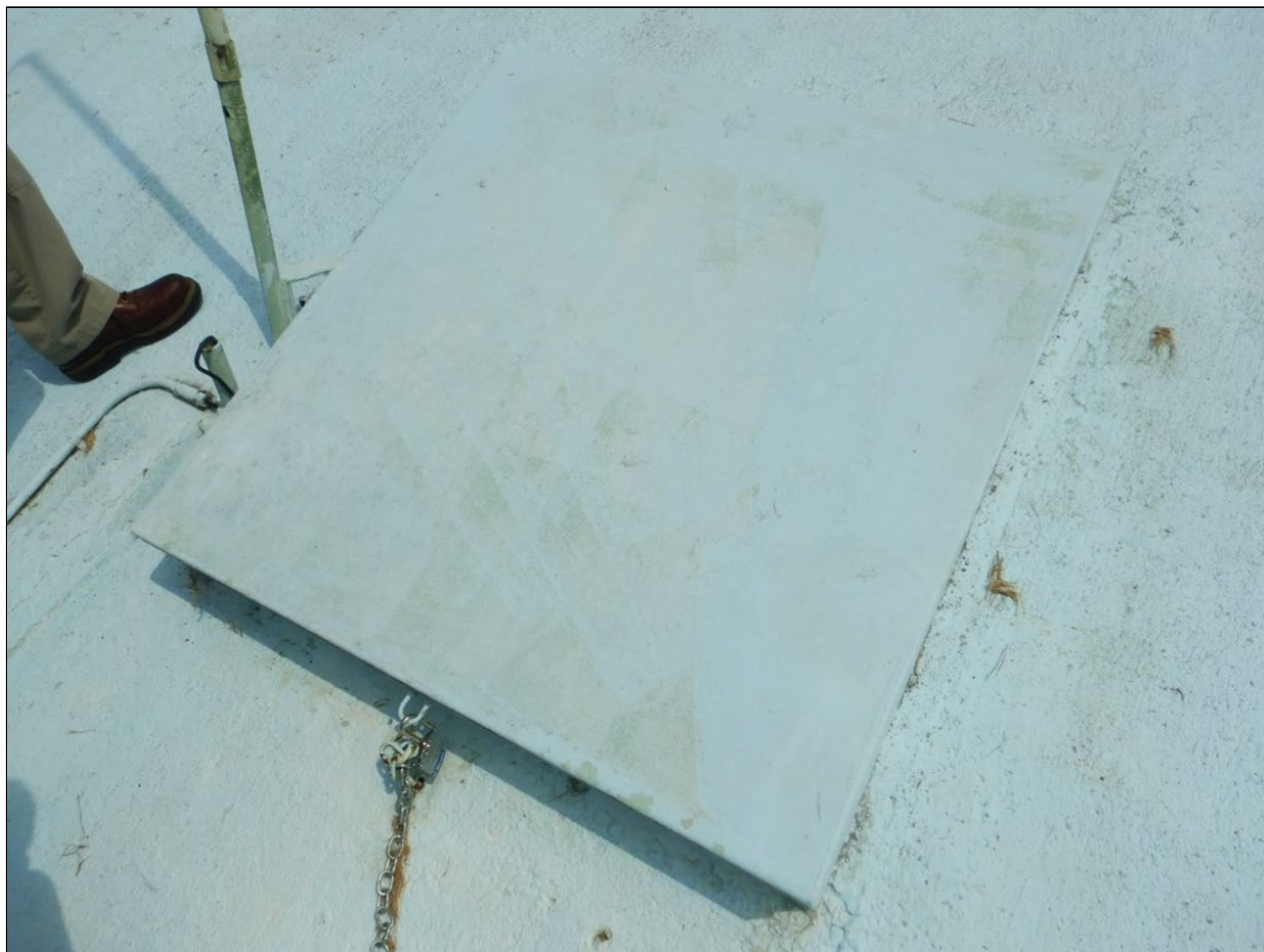
Photograph 23. Front Clearwell, WTP #01 View of the hatchway and lid on top of the Front clear well at WTP #01. The hatchway was locked when the EPA Inspection Team arrived, and this picture was taken after the operator unlocked the lid.
