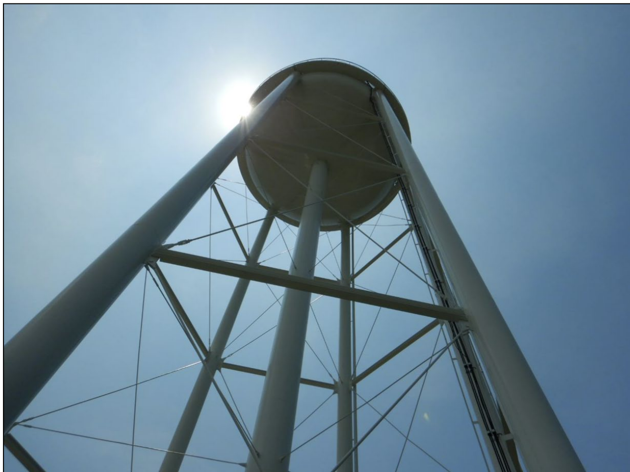
Photograph 35. 16 th St. Water Storage Tank View of the 300,000-gallon elevated 16 th St. Water Storage Tank.
