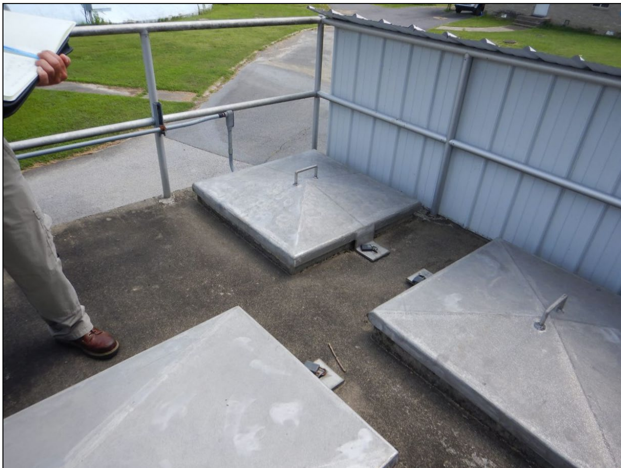
Photograph 21. Backwash Water Holding Tank, WTP #01 View of the hatchways and lids leading to the backwash water holding tank. This tank stores water that is filtered but not chlorinated, and the water is used for backwashing Filter Nos. 3-6. The lids were loosely fitted over the hatchways, and there were no gaskets in the hatchways.
