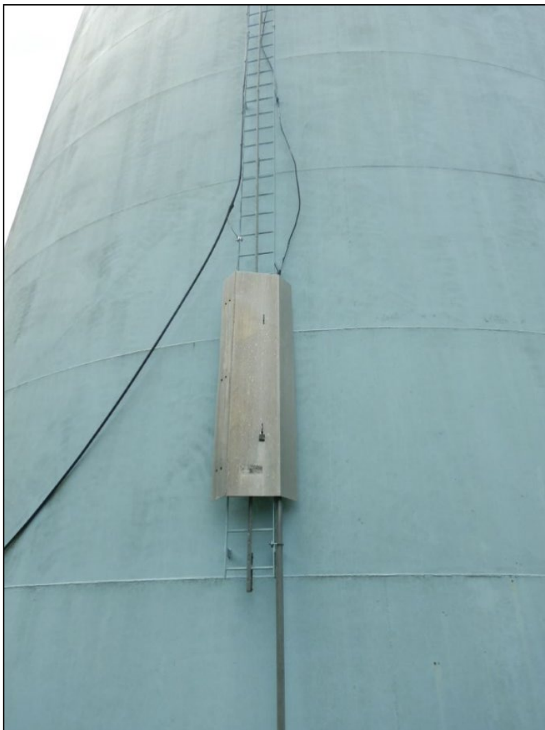
Photograph 32. 26 th St. Water Storage Tank View of the 1,000,000-gallon 26 th St. Water Storage Tank. The bottom rungs of the tank ladder were removed, and there was a locked security shield covering the lower rungs.
