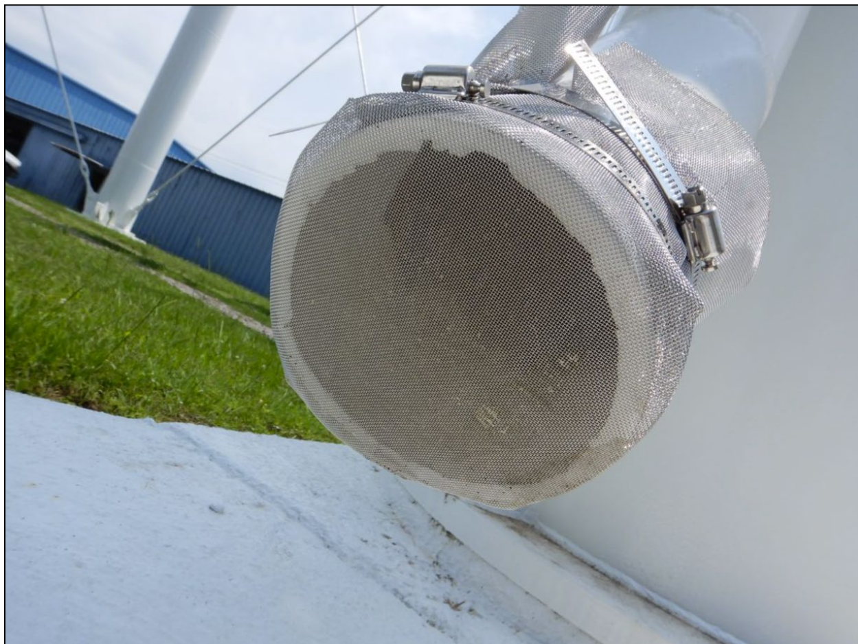
Photograph 38. Overflow Pipe, 16 th St. Water Storage Tank View of the end of the 16 th St. Water Storage Tank overflow pipe. The opening was covered by a mesh screen.
