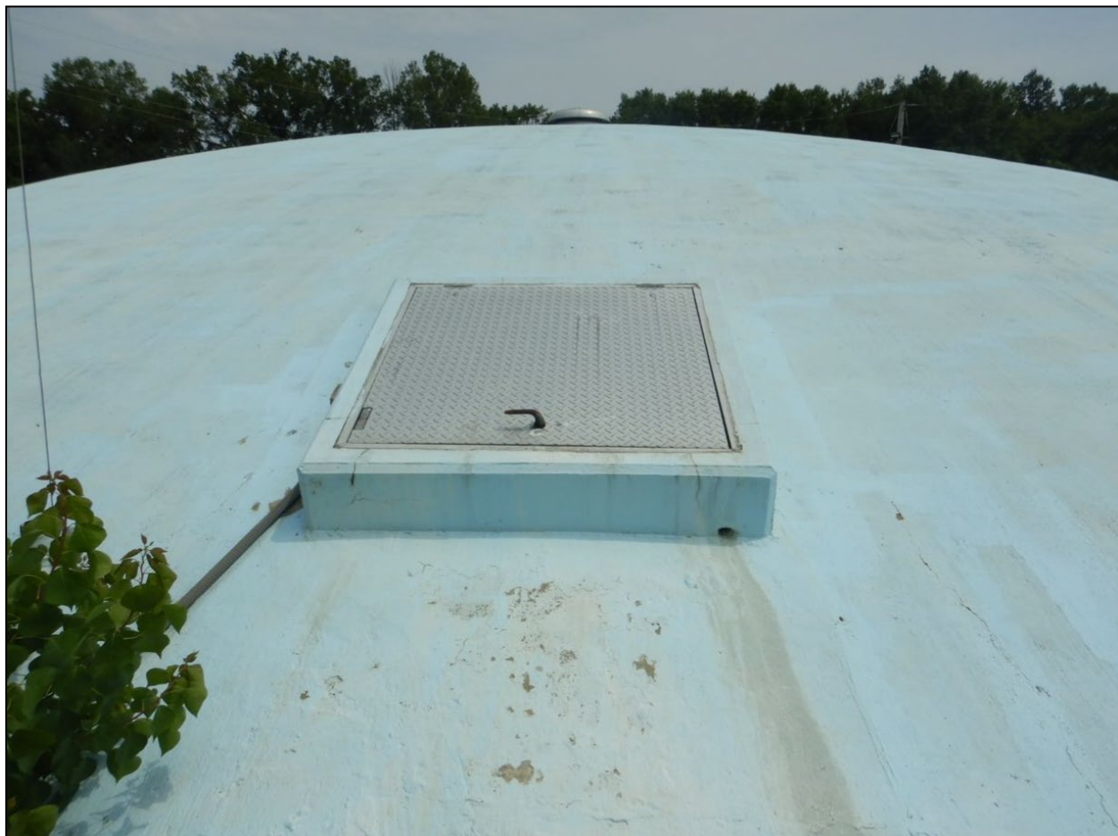
Photograph 27. Back Clearwell, WTP #1 View of the closed hatchway leading to the Back clear well.
