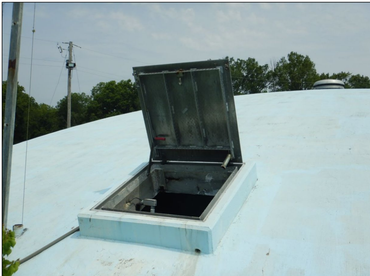
Photograph 26. Back Clearwell, WTP #1 View of the hatchway leading to the Back clear well. The hatchway was elevated, and the rim beneath the lid contained drainage.
