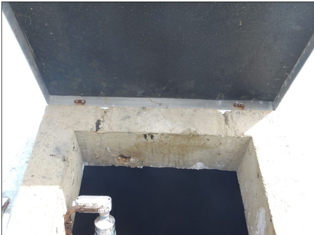
Photograph 24. Front Clearwell, WTP #01 View of inside of the hatchway on top of the Front clear well. The hatchway opening was elevated, and the lid was a shoebox lid which fit around the outside of the hatch.
